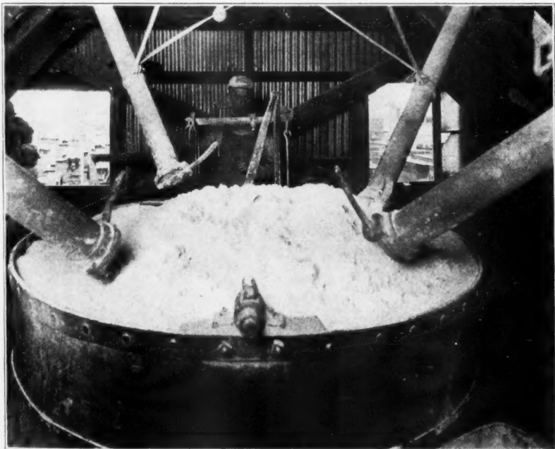
Stucco Mixing Hopper Resting on Scales
